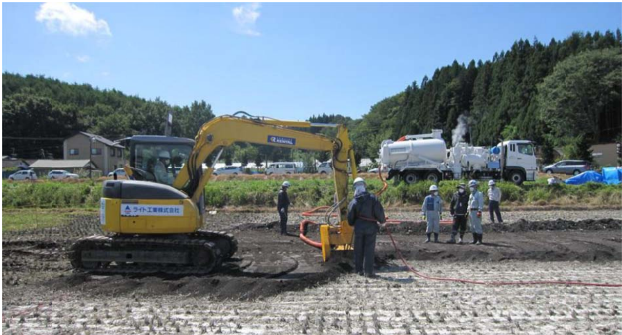
Figure 3: Testing top soil removal after using soil hardener (Courtesy of MAFF-JAEA-NARO).
