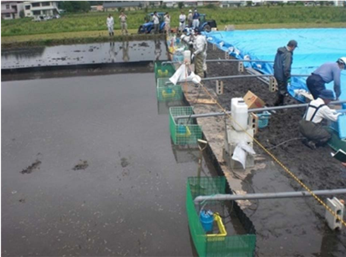
Figure 6: Draining suspended soil from paddies as a remediation option. (Courtesy of MAFF-NARO).
